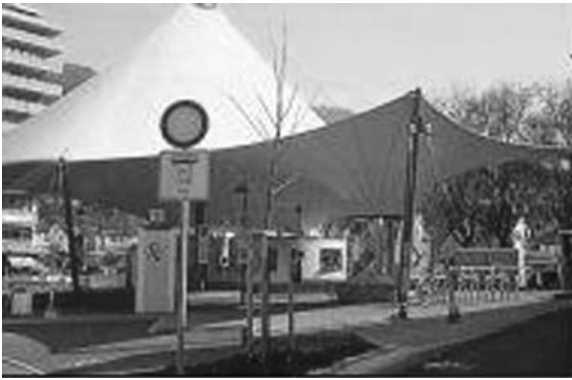
18.25 Railway and bus stations architectural membranes [65].
